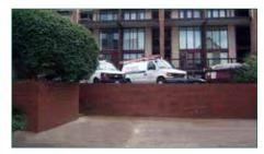
The brick retaining wall in the lower courtyard was cleaned and treated with water repellant.
