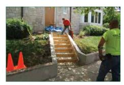
New concrete steps were installed from the door at the west side of the house down to the public sidewalk.
